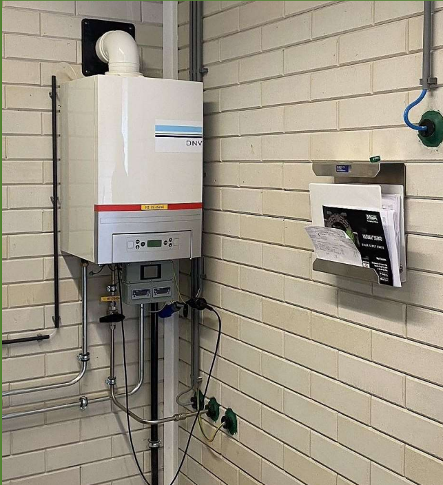
Hydrogen boiler operational since May 2021
