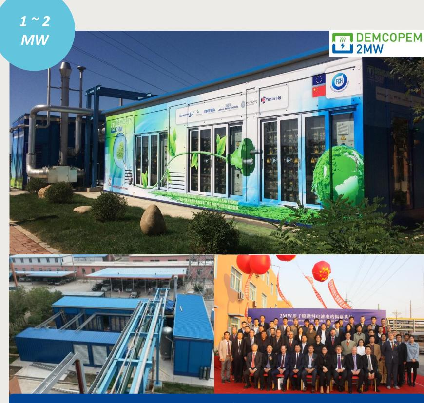
2MW plant at Ynnovate, Yingkou (province Liaoning), China Design, build and operate a 2 MW power generator, with full integration of heat and power with an existing chlorine production plant. Fully automated way of operation + remote control
